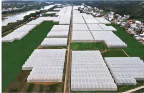
Multi-span Film Greenhouse
